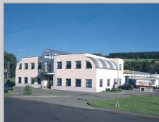
production of cogeneration technology in Hořovice
